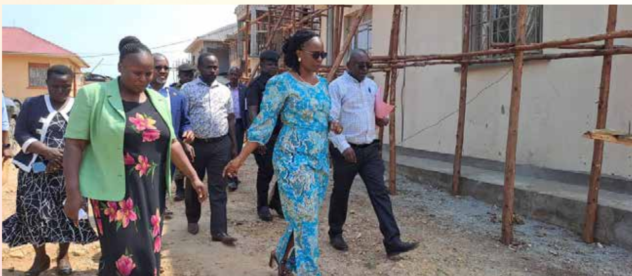
Deputy IGG Mrs. Anne Twinomugisha Muhairwe with technical staff from IG conducting spot check on a project being implemented in one of the Local Government.
