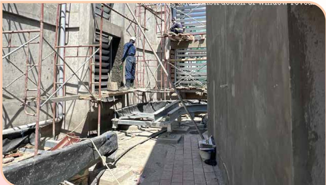
The ongoing construction of the IG Headquarter building
