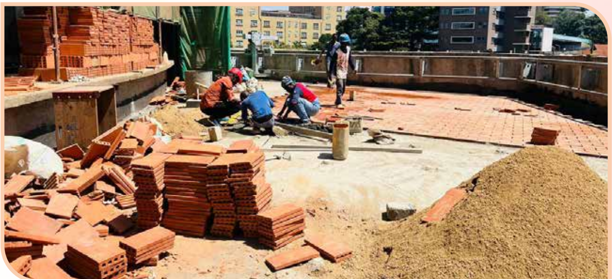
The ongoing construction of the IG Headquarter building
